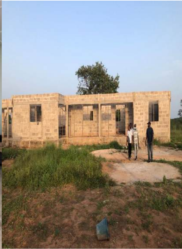
CONSTRUCTION OF 1 NO. 3 UNIT CLASSROOM AT SORI 2
